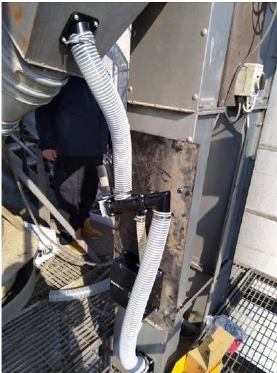
Example of Dosing Auger and Sensor installation
